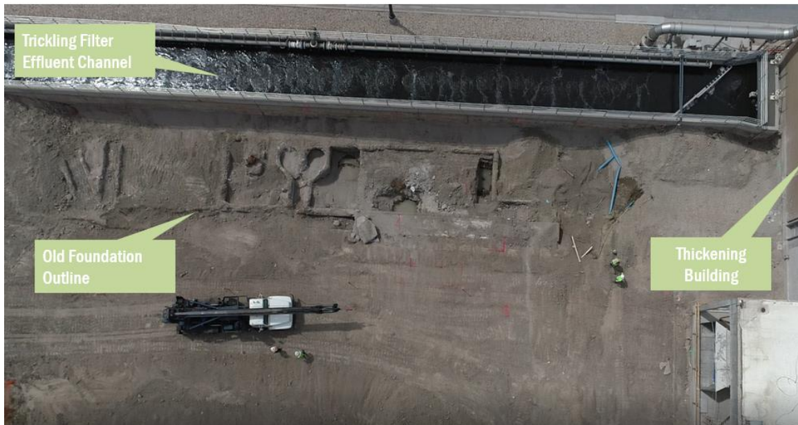
Overhead View Looking South Towards the TF Effluent Channel
