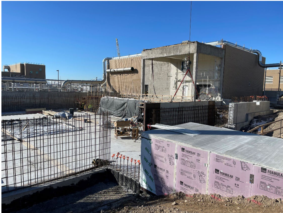
View looking S/W at the Future Straining Building and N/S Tunnel
