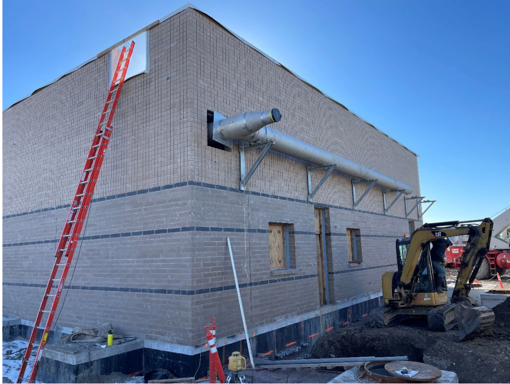
View looking S/E at the West side of the SSN Building
