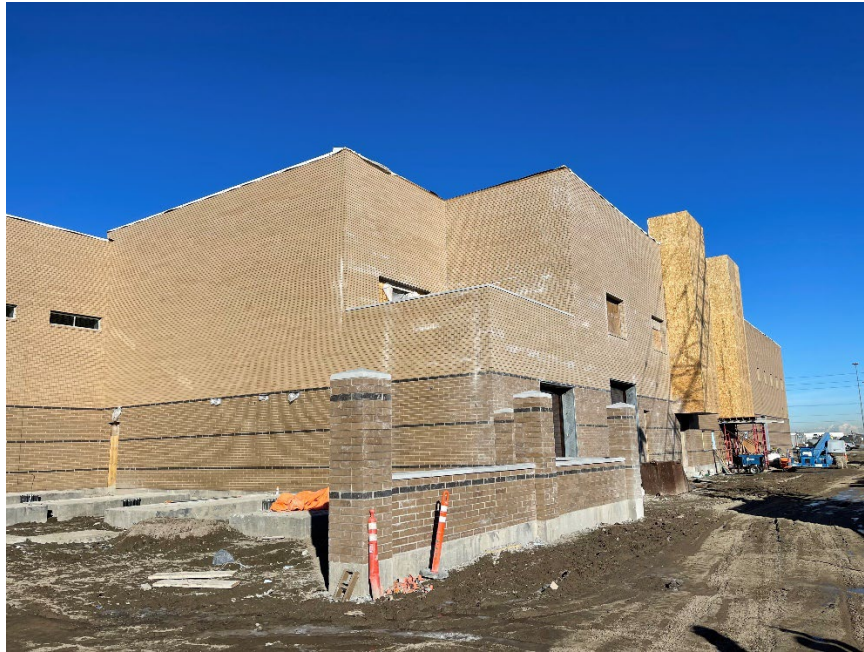
View Looking N/W at the S/E corner of the Blower Building
