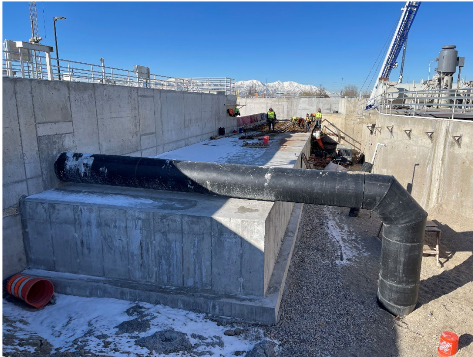
View Looking West at the North end of the Anaerobic Basin
