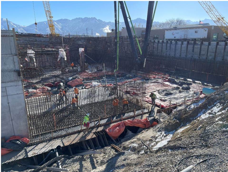
View looking E/SE at Aeration Concrete Slabs & Wall Reinforcement
