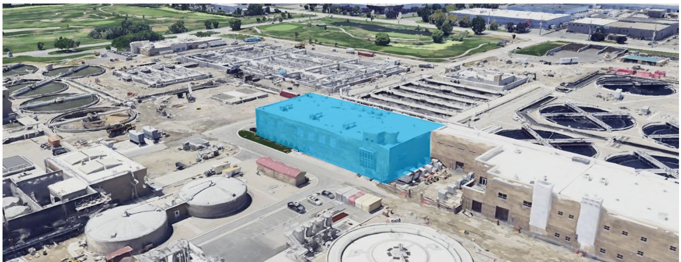
Figure 1 – Power Generation Building (shaded blue)
